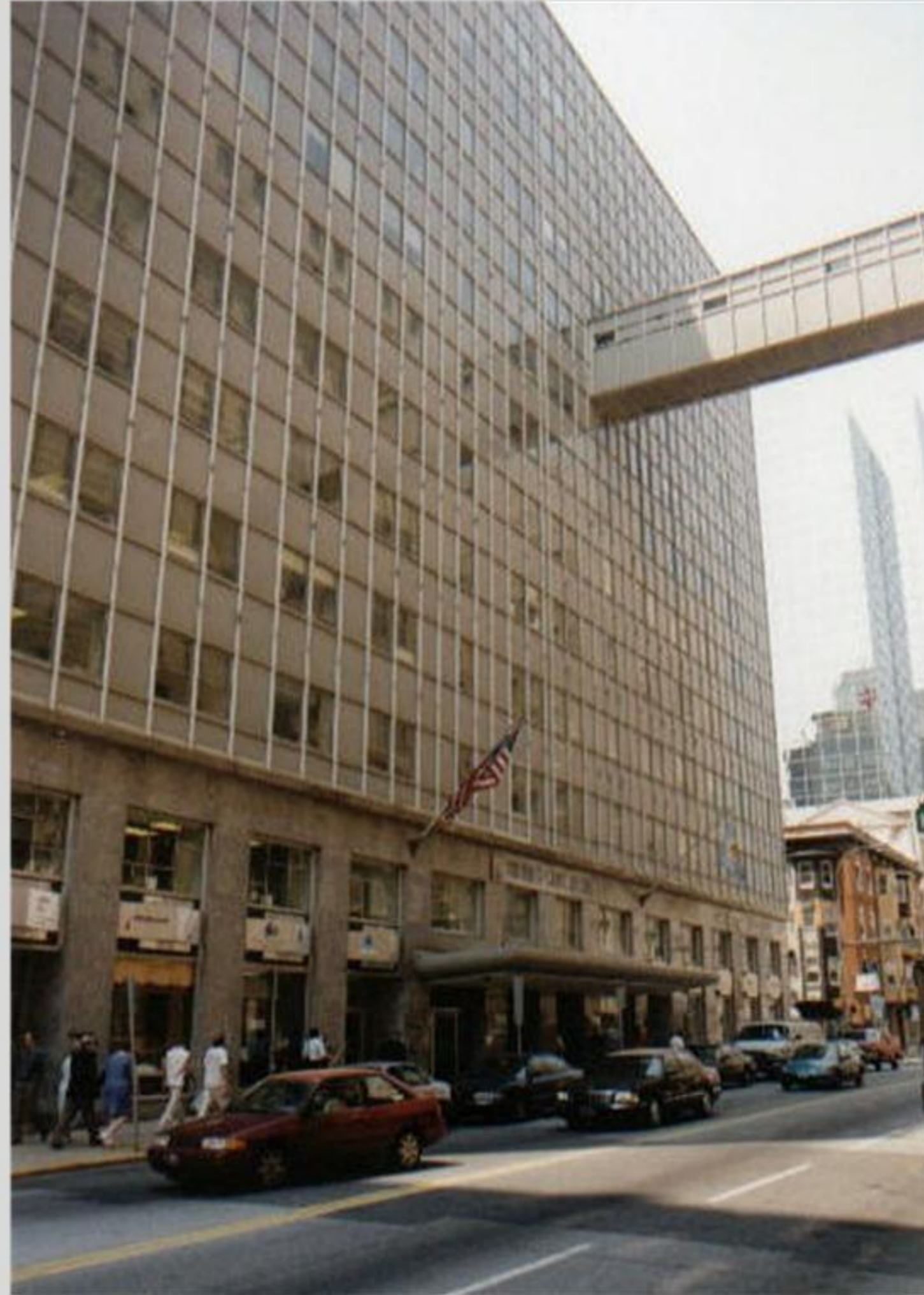
Community Service Building Wilmington, DE
