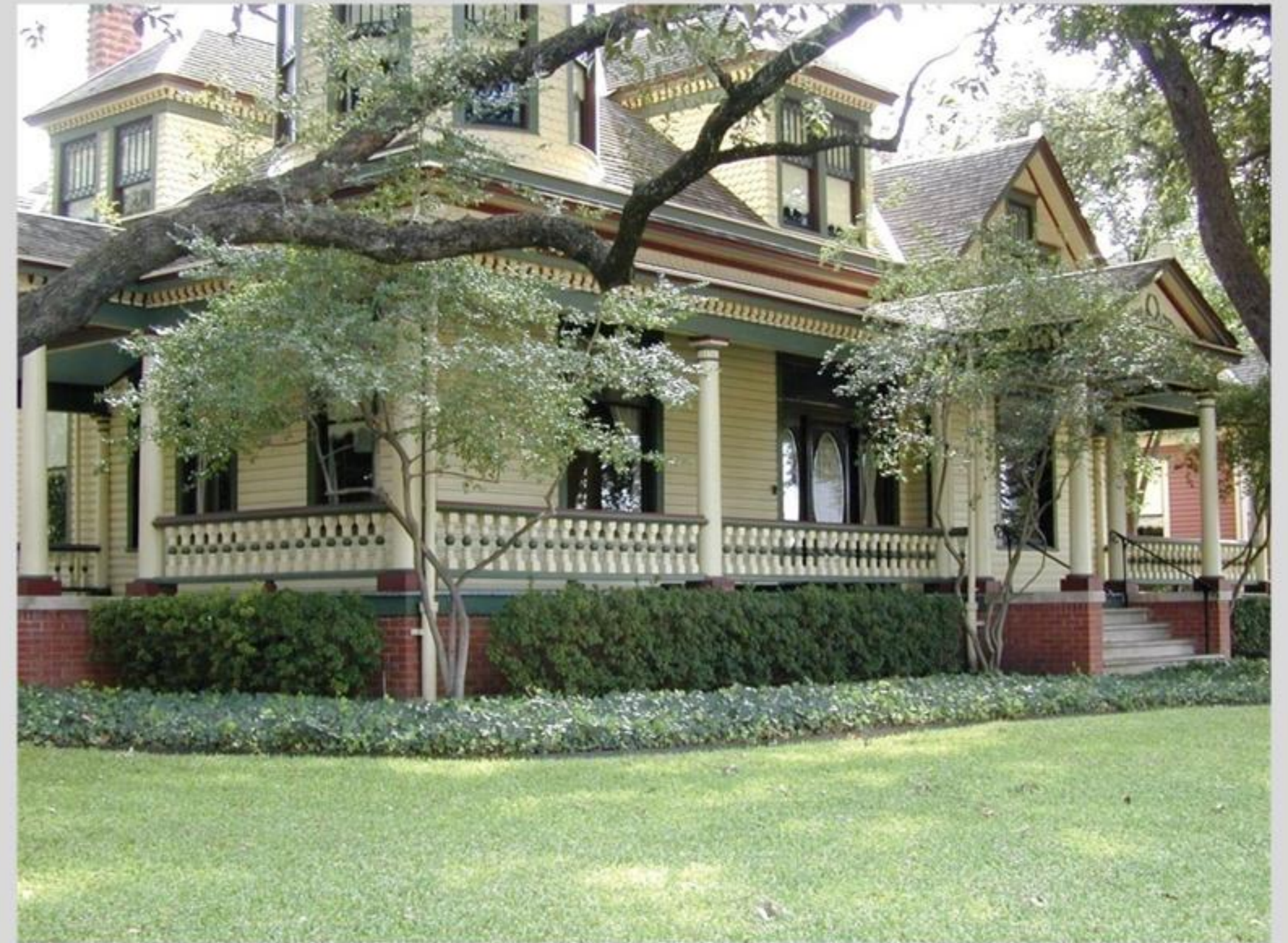
Wilson Historic District Dallas, TX
